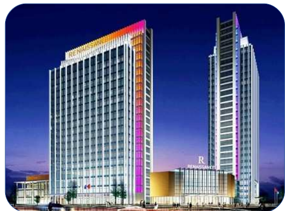
Nanjing Jinao Tower
